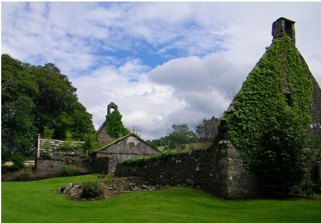
Old Dailly Church had two belfries, both visible in this photo.
